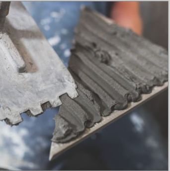
Cement Laying On Tile
