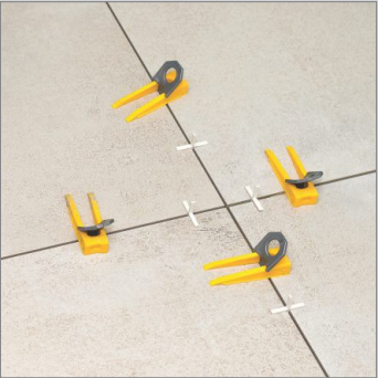
After Lavelling Process Leave Int For 8-10 Hrs.
