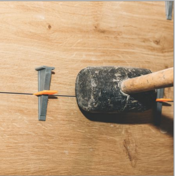
Remove Wedges Ones It Dry
