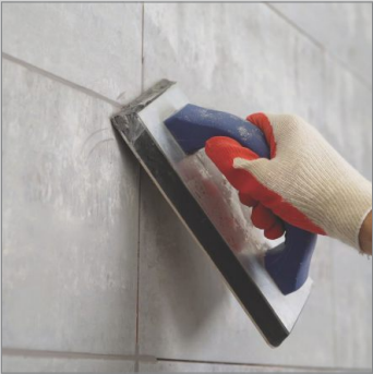
Joint Grouting
