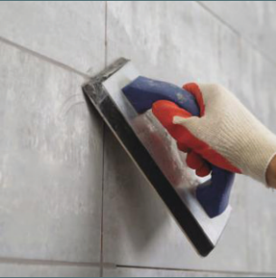
Joint Grouting
