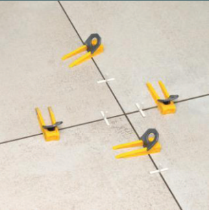
After Lavelling Process Leave Int For 8-10 Hrs.
