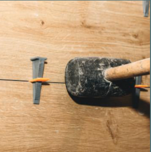
Remove Wedges Ones It Dry
