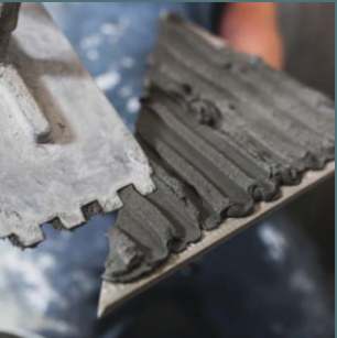
Cement Laying On Tile
