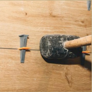
Remove Wedges Ones It Dry
