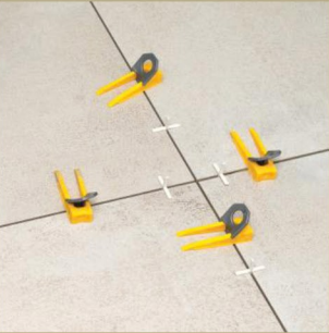
After Lavelling Process Leave Int For 8-10 Hrs.
