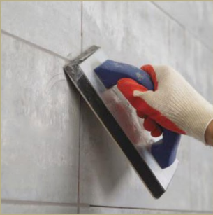
Joint Grouting
