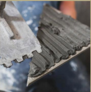
Cement Laying On Tile
