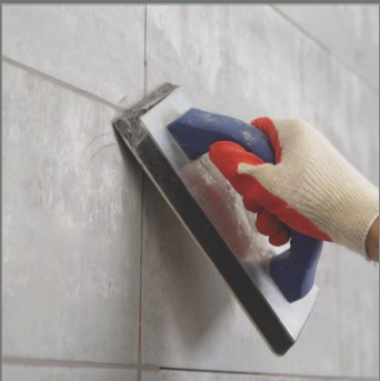
Joint Grouting
