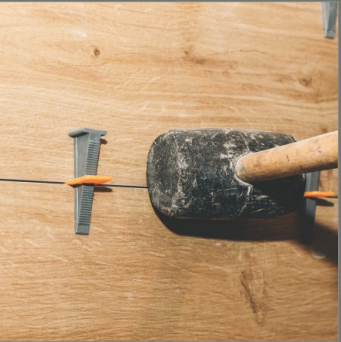
Remove Wedges Ones It Dry
