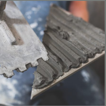
Cement Laying On Tile
